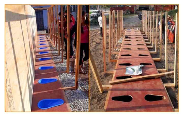
venues. We discovered a revolutionary idea to use sawdust in conventional pit latrines to conceal foul smell, then used the same idea with an enhanced form of pit latrine called trench toilet, where instead of pit we dig a trench to accommodate multiple toilets.
