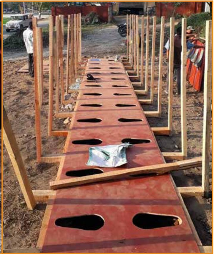
venues. We discovered a revolutionary idea to use sawdust in conventional pit latrines to conceal foul smell, then used the same idea with an enhanced form of pit latrine called trench toilet, where instead of pit we dig a trench to accommodate multiple toilets.
